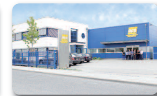
RINGSPANN RCS GmbH, Germany Plant Remote Control Systems
