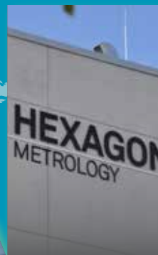
New production hall for ultra-high accuracy CMM's in Wetzlar, Germany
